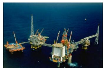
Figure 1: The Sleipner natural gas drilling platform. CO2 is separated from the gas and reinjected to a saline aquifer. (www.statoil.com)
